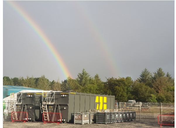
The two tanks containing the deep geothermal water from GEL's well.
